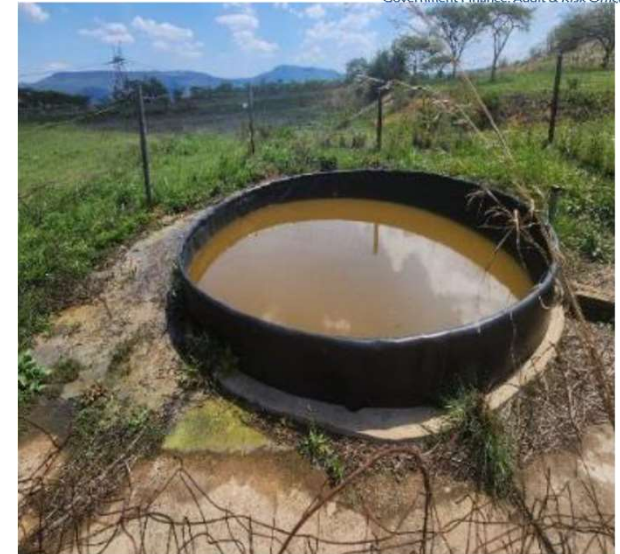
Leachate Pond 1 which had evidence of an overflow of leachate spilling into the environment.
